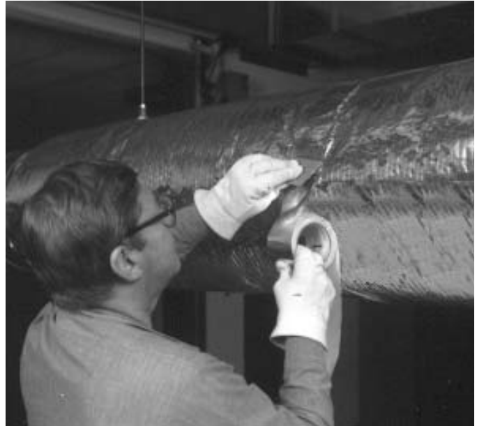
Fig. 22. Fibrous glass duct wrap may be installed on round, oval, or rectangular ducts after joints have been tightly sealed
