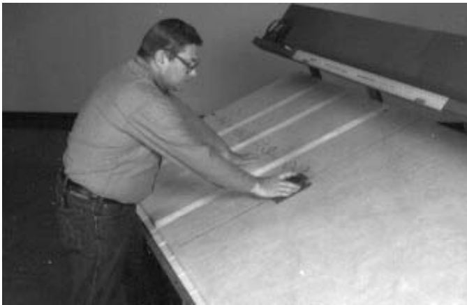
Fig. 10. Hand grooving fibrous glass duct board
