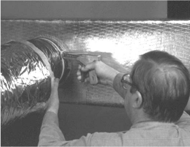
Fig. 31. Applying plastic closure strap to flexible duct
