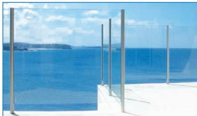
Figure 6 - Structural Balustrade B: Non-compliant above 1 metre fall height. (Source: www.eglasame.com )
