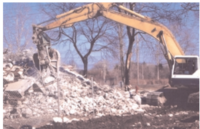
Fig. 5-25. Heavily reinforced concrete is crushed with a beamcrusher. (69779)
