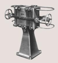
Alfa Laval supplied the first plate heat exchangers to the dairy industry in 1931. Plates were 5-10 mm thick with a milled pattern, compared with 0.4 mm today. In developing our range of plate heat exchangers, we have focused on cost-efficiency.
