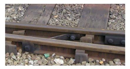
Fig 1 Switch rail anchor on a BH turnout
