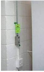
These photos are examples of manual activators that should be used if the automatic extinguishing system fails to activate. This device should be installed away from the cooking surface, next to an entrance/exit for the kitchen. Kitchen staff should be aware of this manual activator and trained on its use. Also note the inspection tag. Many fire service companies will place these tags on the manual activator to indicate current servicing.
