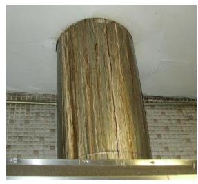
This photo shows ductwork from a cooking area that has a heavy accumulation of grease. Maintaining and cleaning the hood and ventilation system is crucial, as the buildup of grease can become a serious fire hazard. The hood and ventilation system should be inspected and cleaned by a certified contractor every six months.
