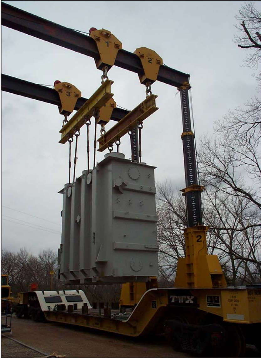
Figure 5.6-5 Hydraulic Gantry Lift
