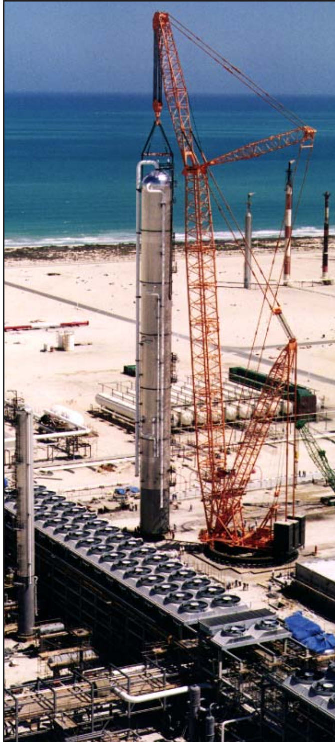
Figure 3.6-2 Ringer Attachment
