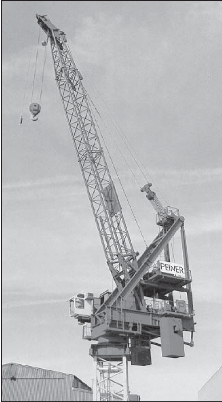
Figure 3.4-2 Luffing Jib Tower Crane
