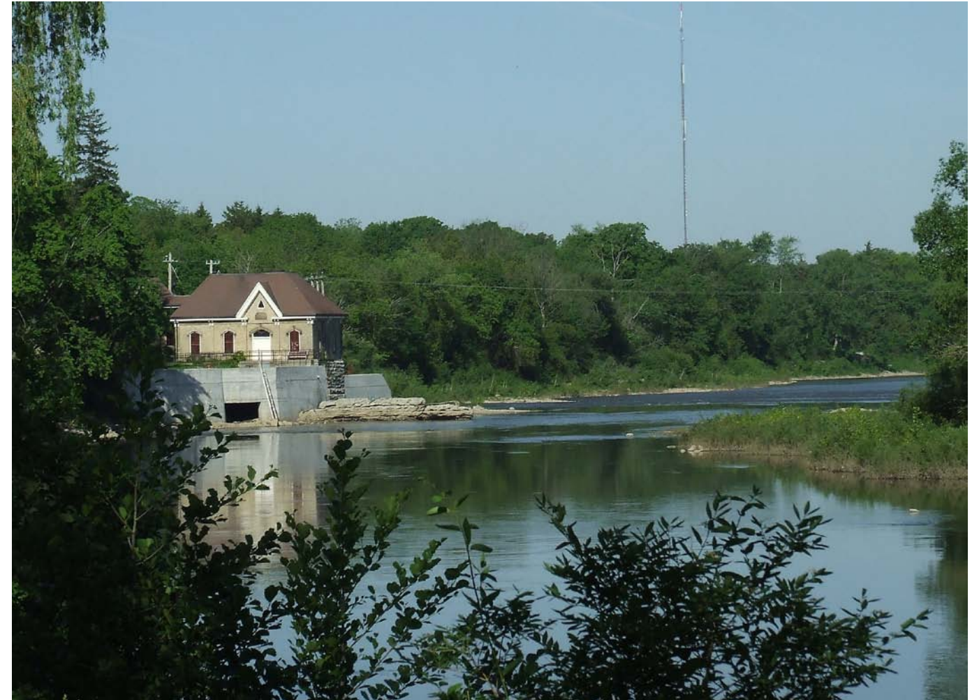
Pumphouse in Springbank Park
