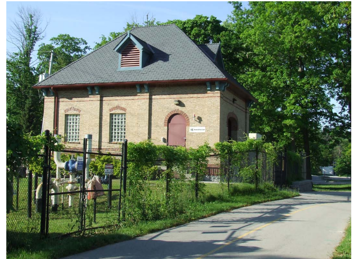
Municipal infrastructure in Springbank Park
