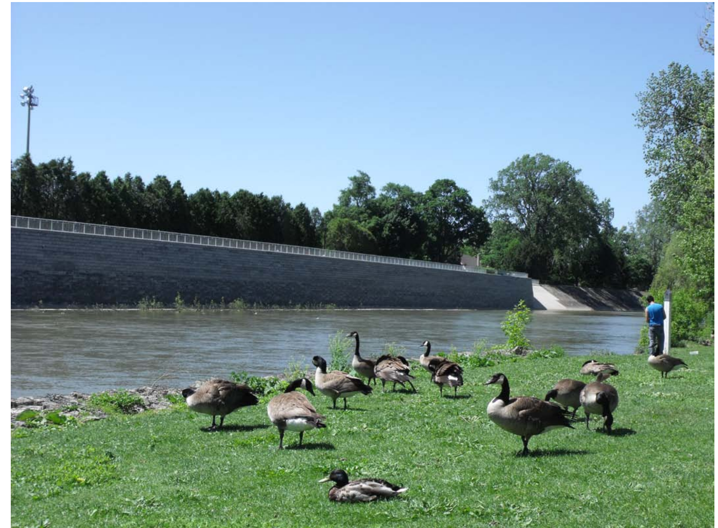
The recently constructed dike located along the west side of the Thames River, opposite Harris Park, won a design award in 2010. The dike protects residents from flooding events.
