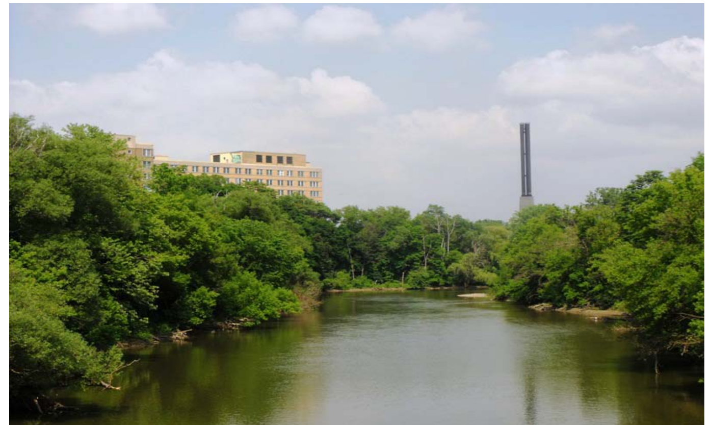
Looking East on the South Branch of the Thames River toward the South Street Hospital Campus
