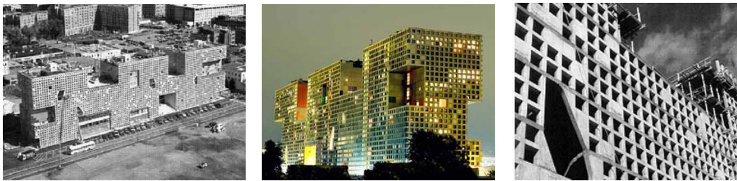
Figure 1. Simmons Hall student residence at MIT. Windows on the facades.
