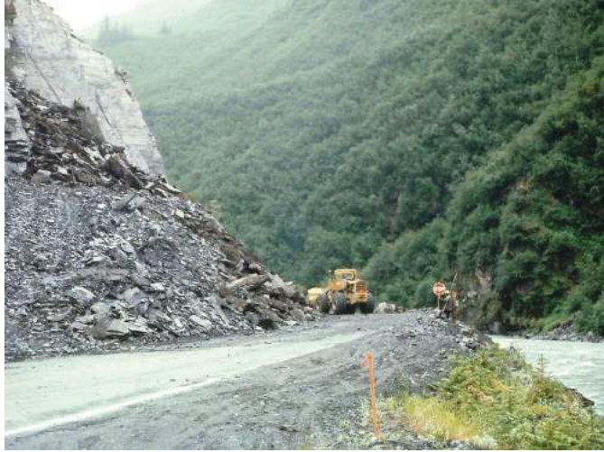
FIGURE 8-3. Weathering weakens rock so that it falls under the influence of gravity.
