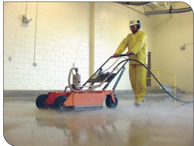
Fig. 7. Waterblasting equipment can prepare horizontal surfaces without damaging the concrete substrate. (IMG25539)
