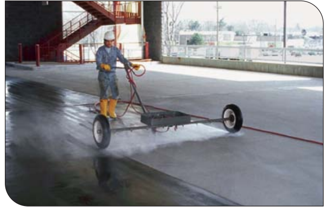
Fig. 9. 100% silane sealer is being applied to a parking garage. (IMG25538)
