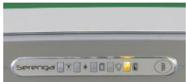
Self-Test exit sign showing green LED for correct performance or amber LED for fault
