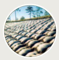
All Fabriform® fabrics are manufactured with 100% continuous multifilament, high-tenacity nylon for stability and resistance to the strong alkalis present in concrete and are woven such that at least 50% by weight consists of textured fibers for optimum filtering characteristics and adhesion to mortar.
