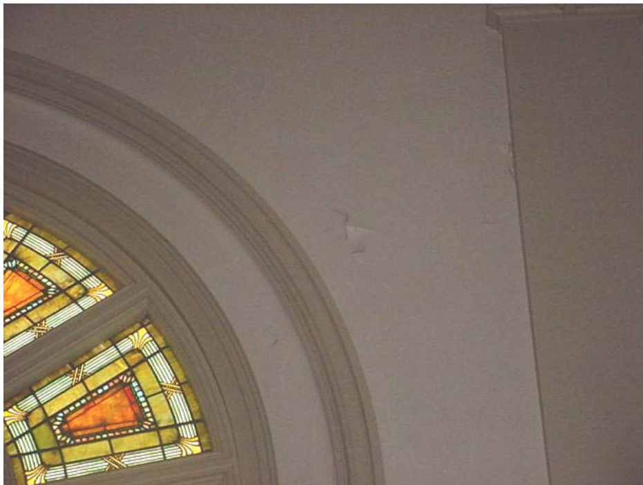
Figure 18. On-site photograph; wall near stained glass window.
