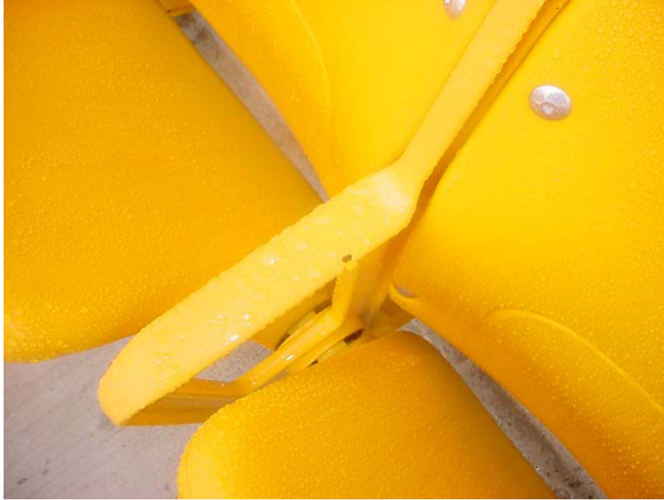
Figure 21. Close-up field photograph of failed touch-up paint on seat standard.
