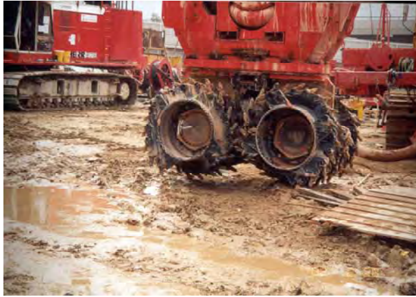
Plate 4.1 A Milling Machine
