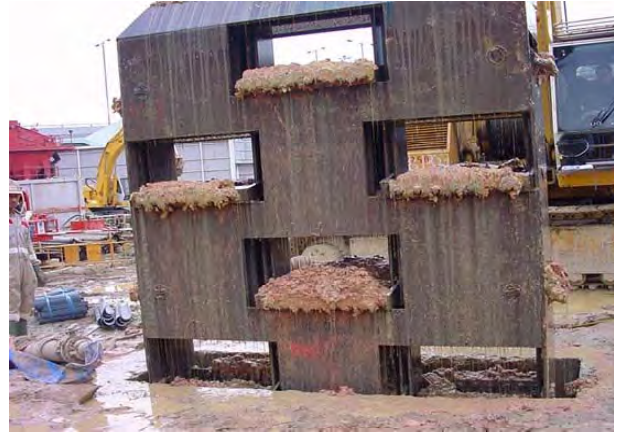
Plate 4.2 A Trench Scraping Unit in Barrette Construction
