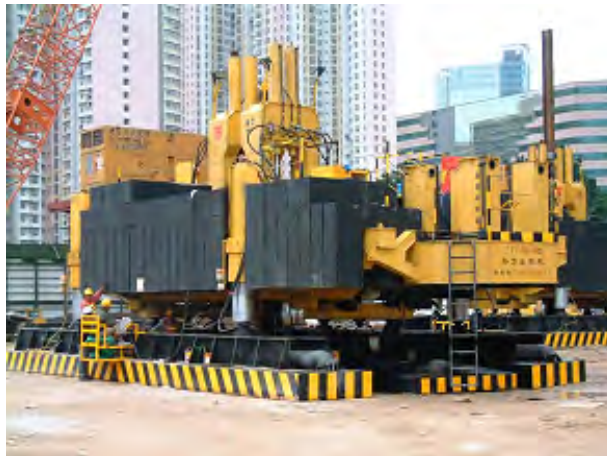
Plate 4.3 – A Pile Jacking Machine
