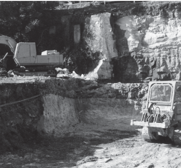
Sudden changes in sub-surface conditions revealed by site excavation.
