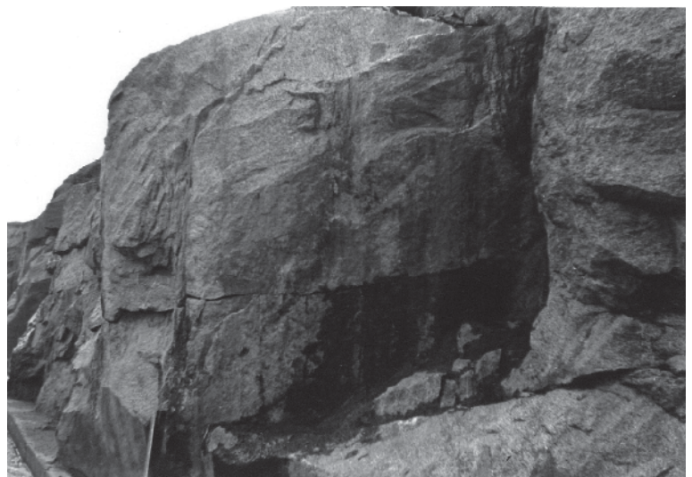
Typical granite country showing boulders outcropping on a hillside. A cutting in granite shows the unevenness usually associated with this rock excavation.
