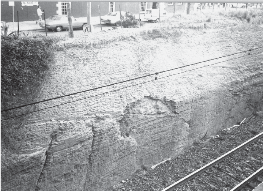
A deep railway excavation in solid shale approximately 100 years old.
