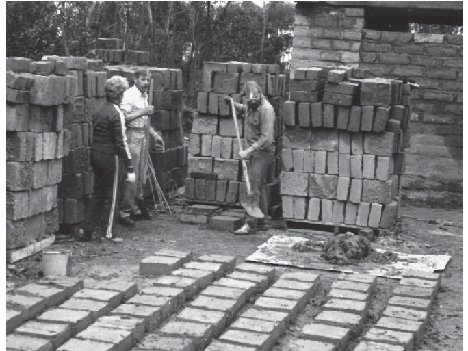
Mud blocks in preliminary drying, stacks and walling. The mix for these blocks contained some cement and was effectively done using a rotating cement mixer.
