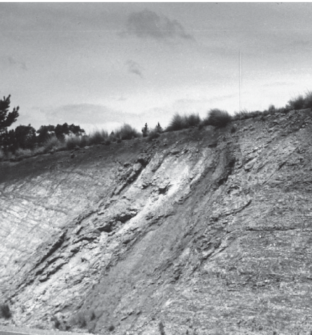
Sudden changes in sub-surface conditions revealed by site excavation.
