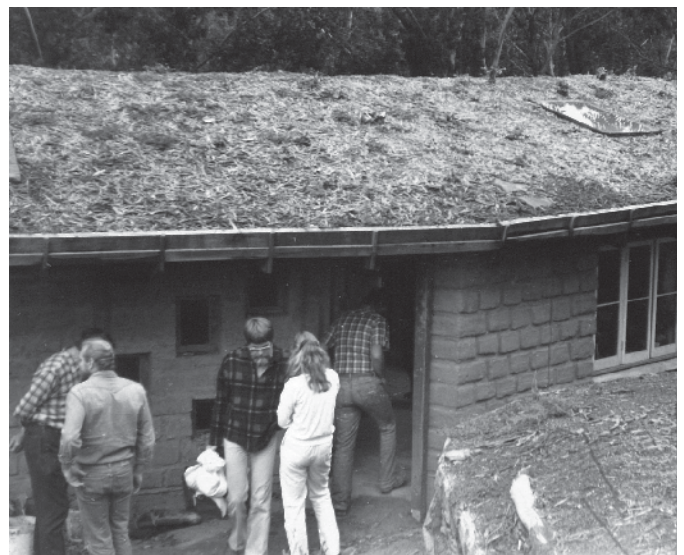
A finished adobe house which also employs an earth-covered roof over a waterproof membrane.
