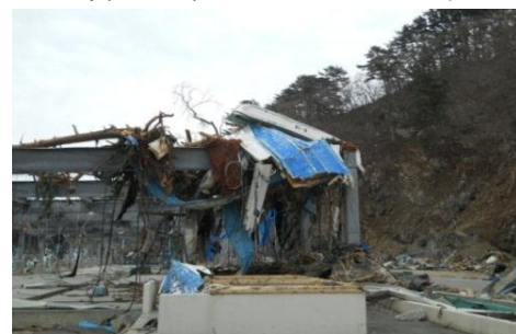
Fish landing facility damaged by the tsunami (Miyako City, Iwate Prefecture)
