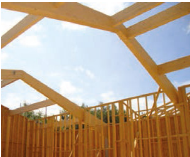
Figure 9 Glulam portal frames
