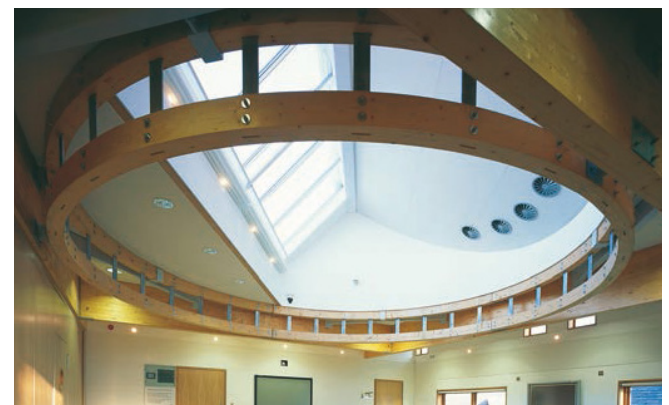
Figure 6 Vertically laminated, curved on plan glulam
