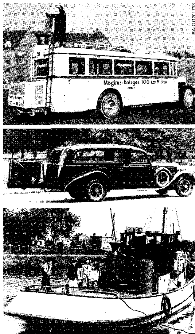
Fig. 2-1. Vehicle gasifiers before 1950 (Source: NAS 1983)
