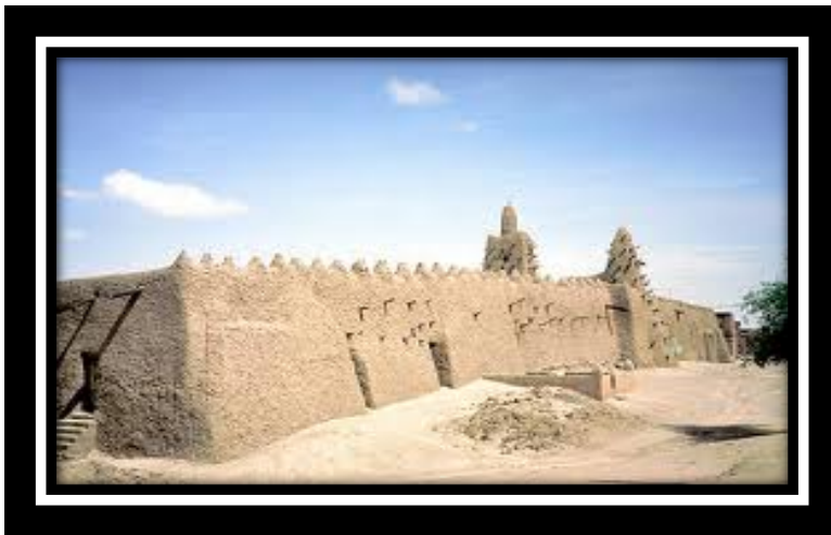
Djingareyber Mosque, in Timbuktu
