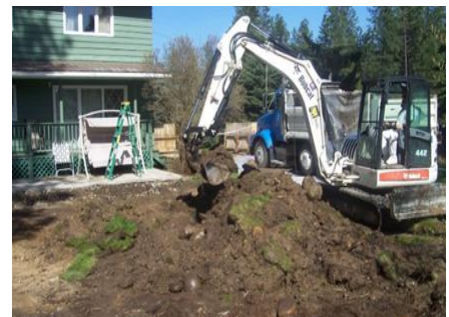
Cleanup at a Libby residential property. (EPA photo)
