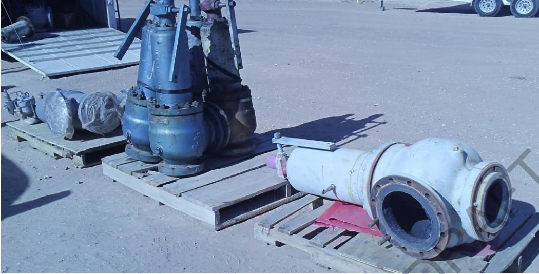
Figure 36 - Improper Storage of Valves
