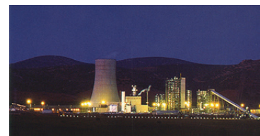
Puertollano IGCC Power Plant
