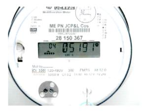
The register index in this case is the "05191". The index is like the odometer in a car. It increases in increments only until it reaches "99999" and then it returns to zero.
