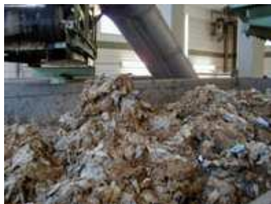
Photo 1: Separated solids (source: Stadtentwässerung Göttingen)
