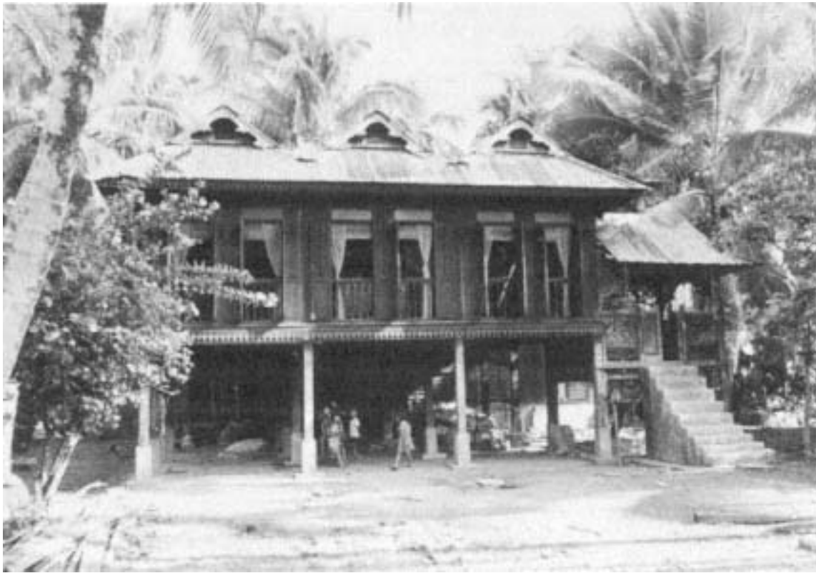
10. House of well-to-do local farmer. Note clapboards, shutters, zinc roof, and veranda.
