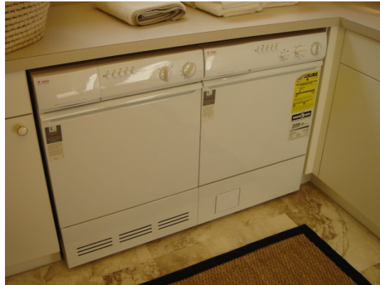
Figure 16. Clothes dryers—Where clothes dryers are installed, they should be unvented condensing units—or if vented to the exterior, a provision for powered make-up air must be made
