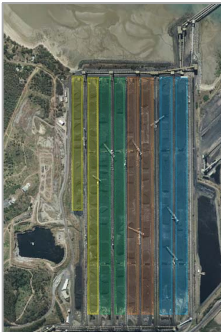
Figure 13: DBCT 7X zonal yard layout incorporating Remnant Management in rows 7 & 8 – (DBCT Management, 2016)
