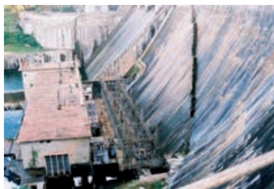
PHOTO 10.1 Power plant at a reservoir Karnataka, India
