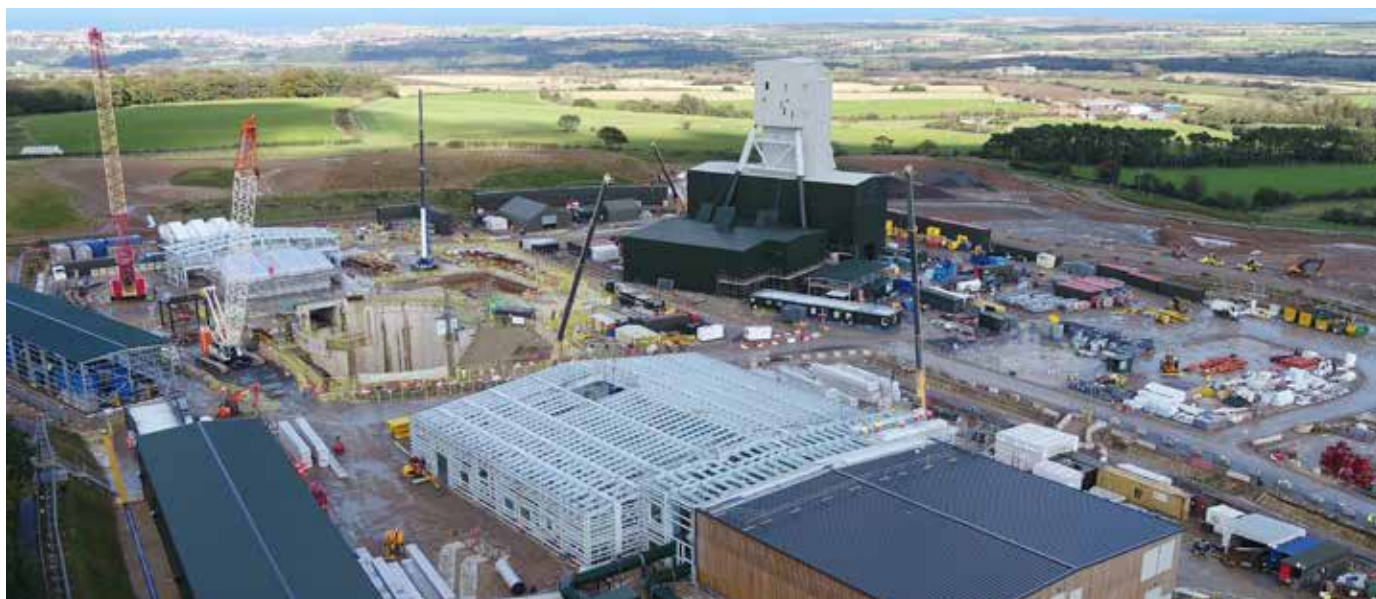
Construction at the Woodsmith project as at October 2020.
