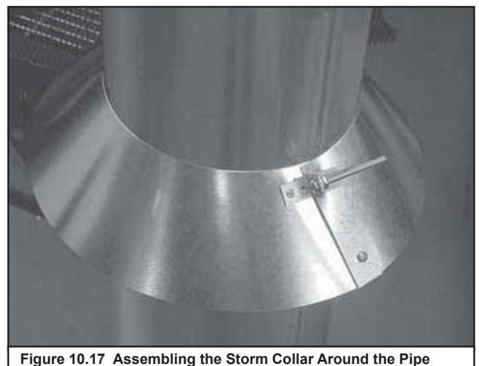
Figure 10.17 Assembling the Storm Collar Around the Pipe
