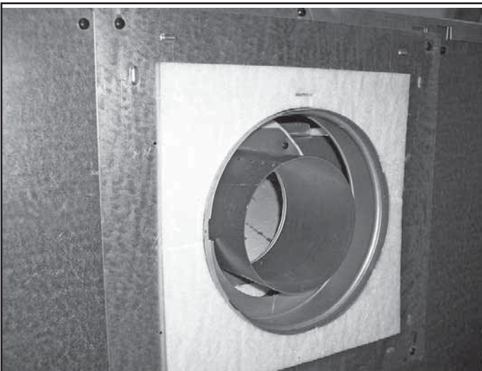
Figure 9.13 Place Insulation over the Cover Plate
