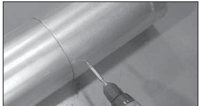
Figure 10.7 Screws into Slip Section
