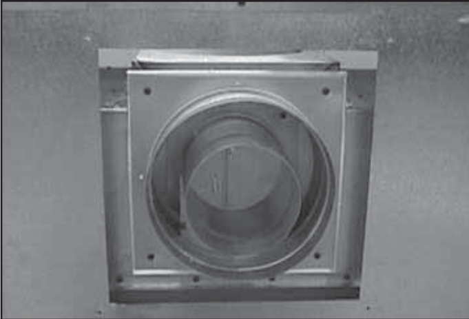
Figure 9.11 Place Outer Collar on Rear of Appliance
