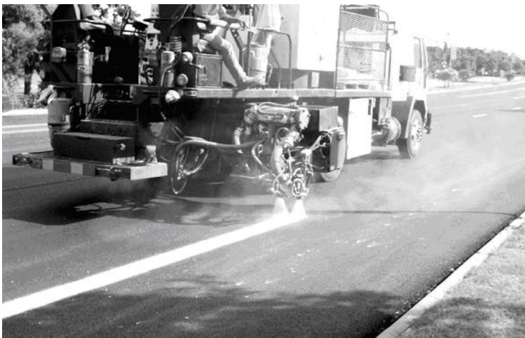
Figure 2-10. Typical sprayed thermoplastic operation.
