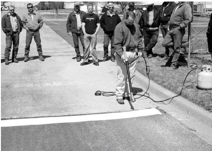
Figure 2-16. Typical preformed thermoplastic application.
