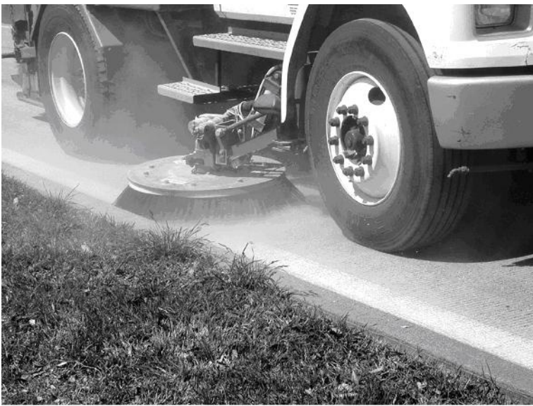
Figure 2-8. Typical brooming operation for surface cleaning prior to striping.
