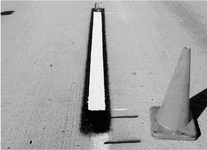
Figure 2-14. Typical bordered-contrast pavement marking for lane line.
