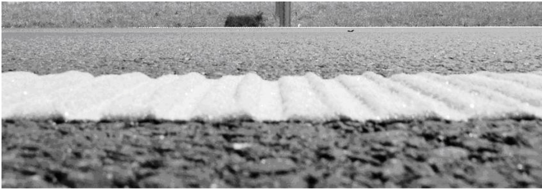
Figure 2-12. Typical inverted-profile thermoplastic marking (profile view).
