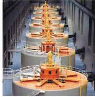
A generator inside a hydroelectric dam uses electromagnetic induction to convert the mechanical energy of a spinning turbine into electric energy.
