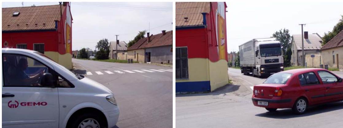
Figure 6-7 and 6-8: Insufficient sight distances
