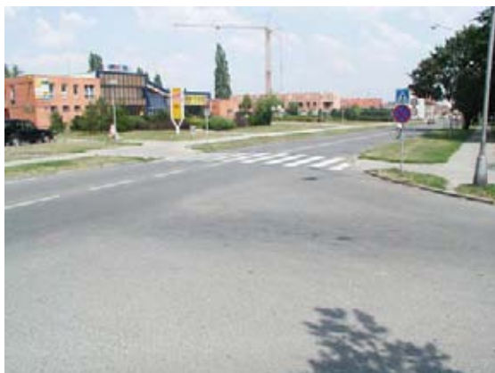
Figure 6-3: Crossing is too long
