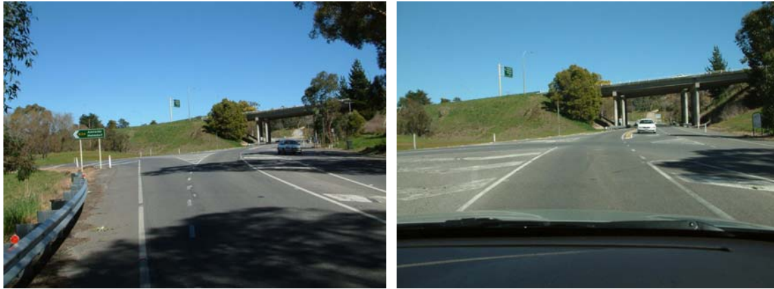
Figure 6-32 and Figure 6-33: Before reconstruction - Looking west
