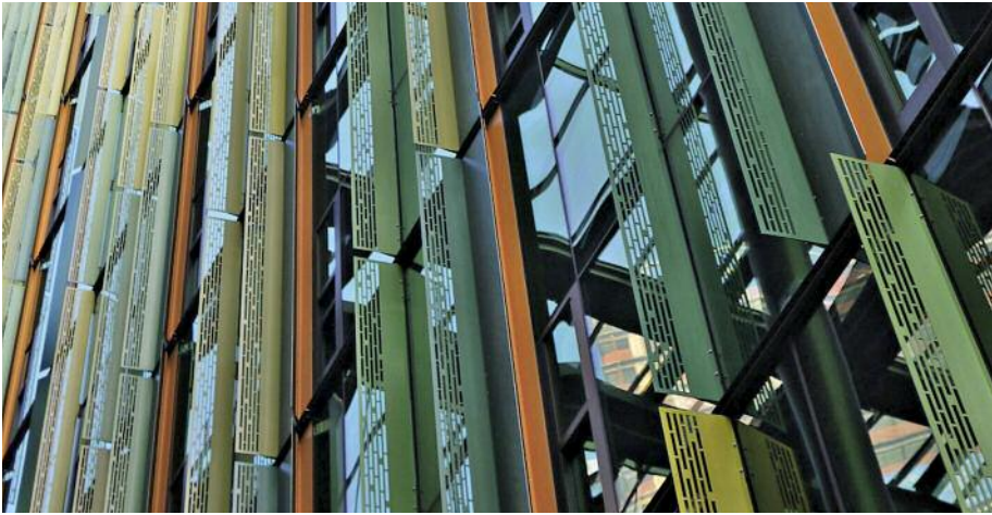
Electrochemically colored stainless steel fins (except orange) on the Doppler Building in Seattle. © IMO A
