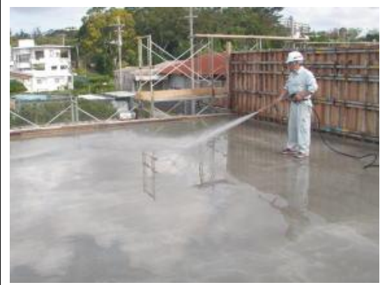
Figure 10-1 Water Curing
