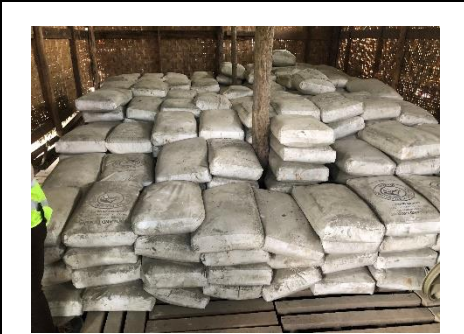
Figure 6.1-2 Recommendable Plan for Storage of Cement Bags
