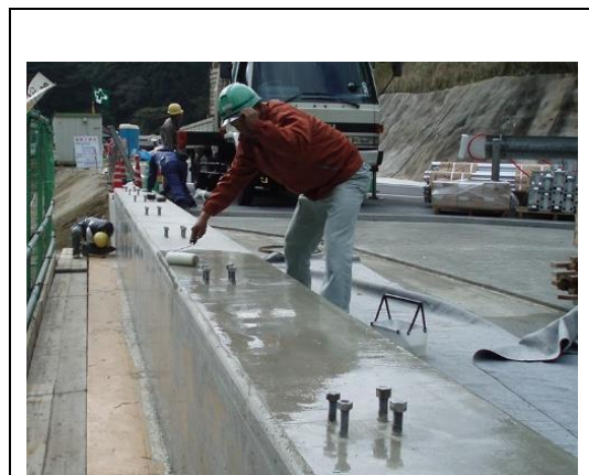
Figure 10.1-2 Liquid Membrane Curing
