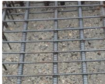
Figure 11.2-3 Completion of Treatment of C.J
