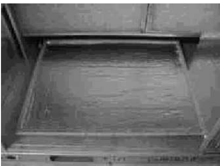
Figure 18: Return Downflow Plenum With Panel
