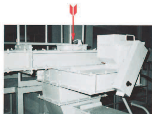
Used for inspection at the cross section between two conveyors
