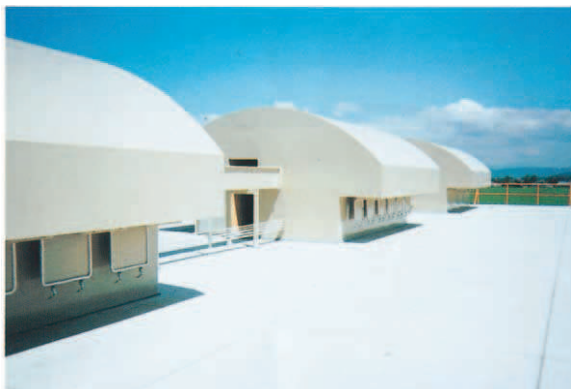
Standard type P4 used as hoods for drying rice paddy
