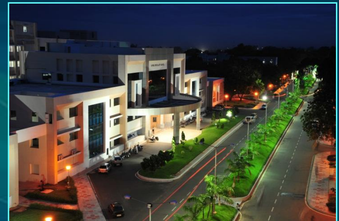
SS Block, JIPMER, Puducherry
