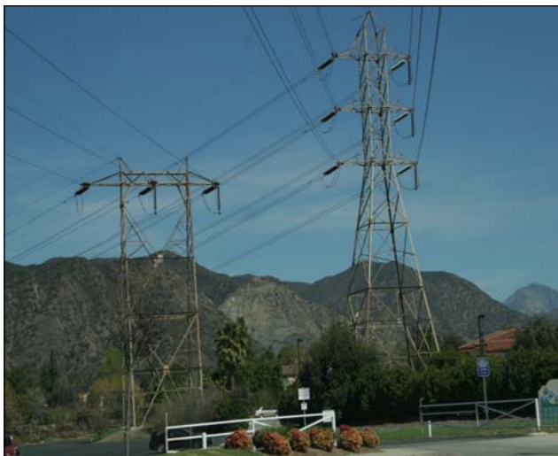
Dead-end towers at a turn in the line. Note the relative sizes of the single-circuit (left) and double-circuit (right) towers.
