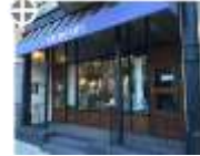
1-story Retail Building
