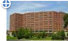
10-story Office Building
