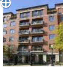
52-unit Apartment Building
