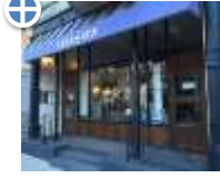
1-story Retail Building
